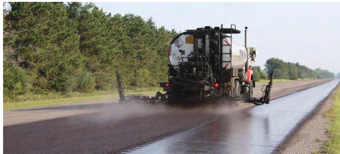
Fog sealing of a chip seal placed on state road.
